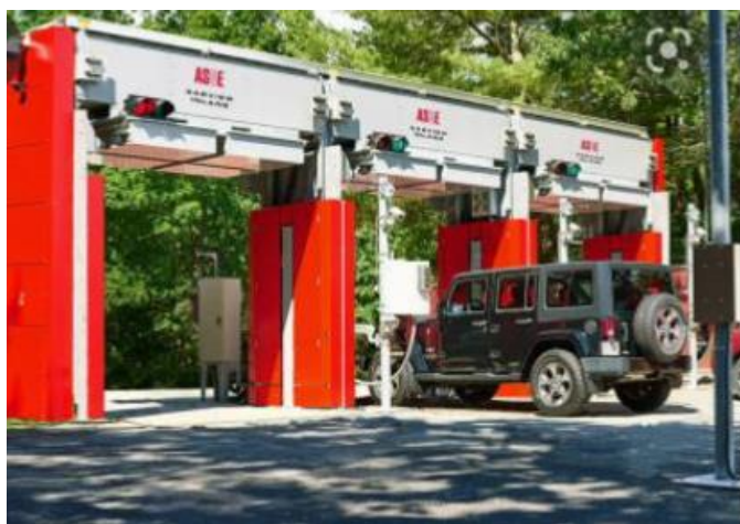
Figure 1: CVIL imaging system installed on the US-Mexico border.
